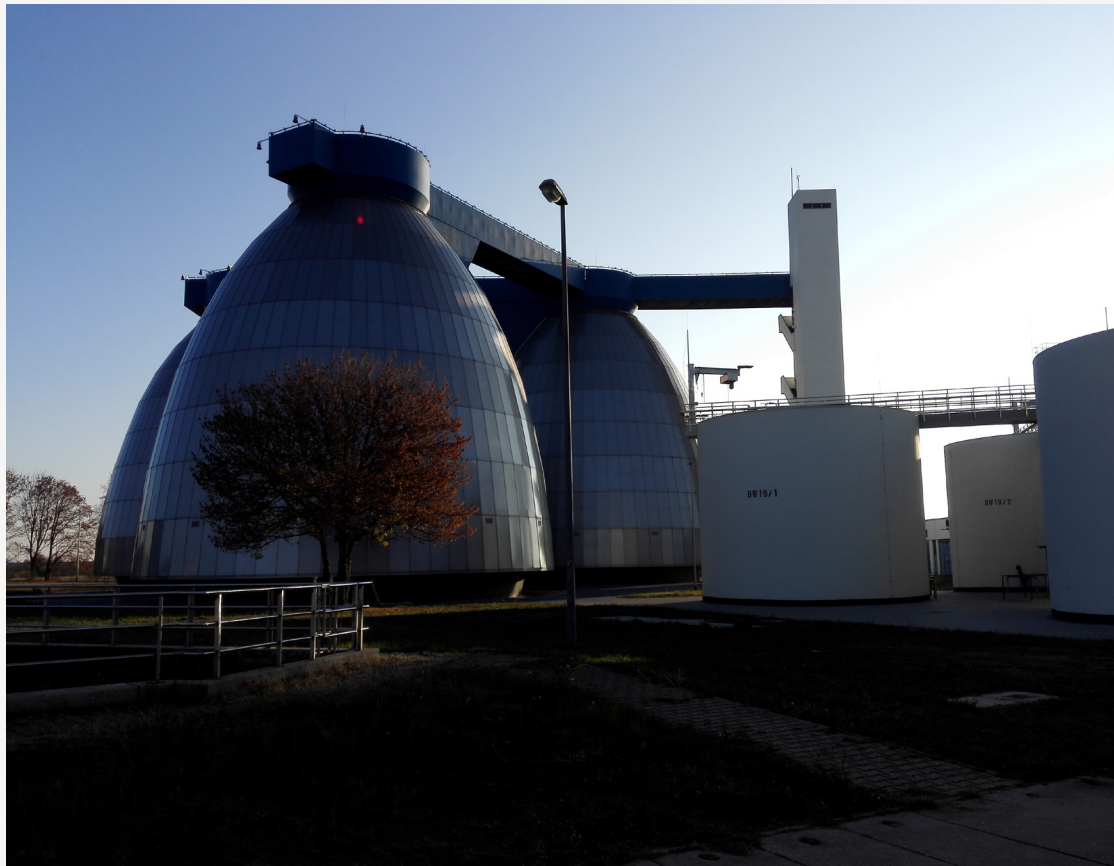
by Bartosz Wilkuzs Sewage plant Mannheim
